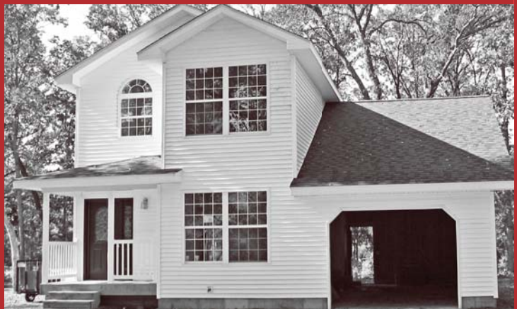
Below: Single family housing developed in the Village of Baldwin.
